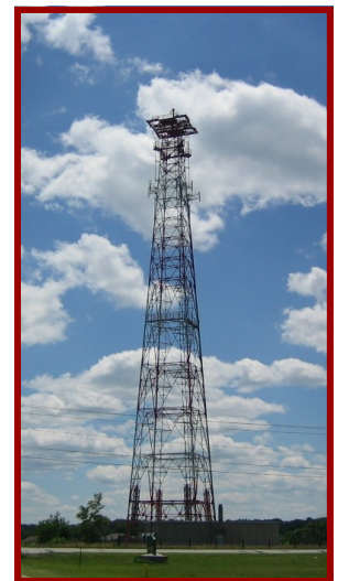
Communications Tower Near Wheatfield
