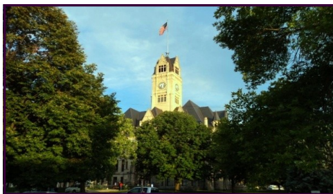
Jasper County Court House in Rensselaer
