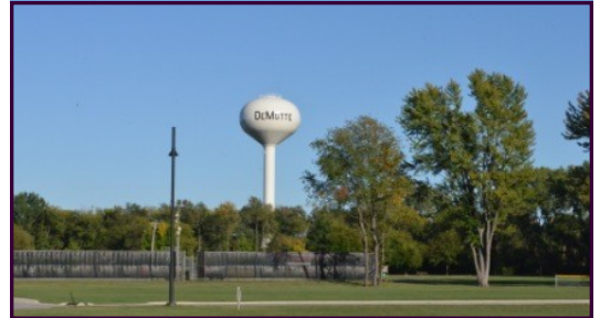
Northern Jasper Regional Water District Tower in DeMotte
